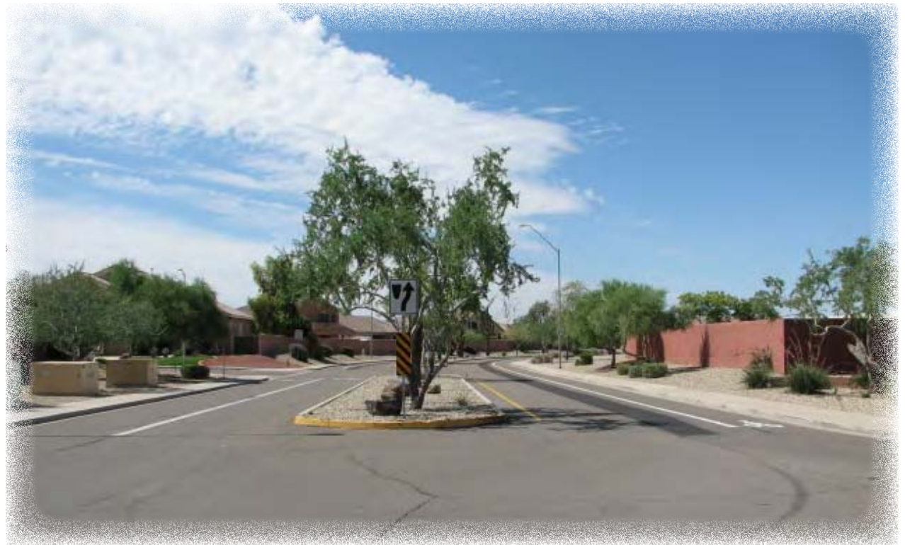
This Complete Streets best practice, from the City of Peoria, demonstrates how a bicycle lane was included by eliminating a vehicle lane. Photo credit: Brandon Forrey.
