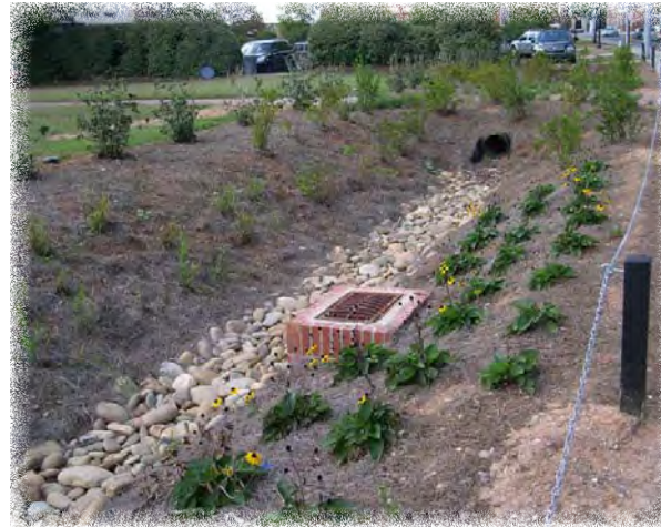
A bioswale reduces storm water runoff and creates a natural filtration system. Photo credit: LIDC
