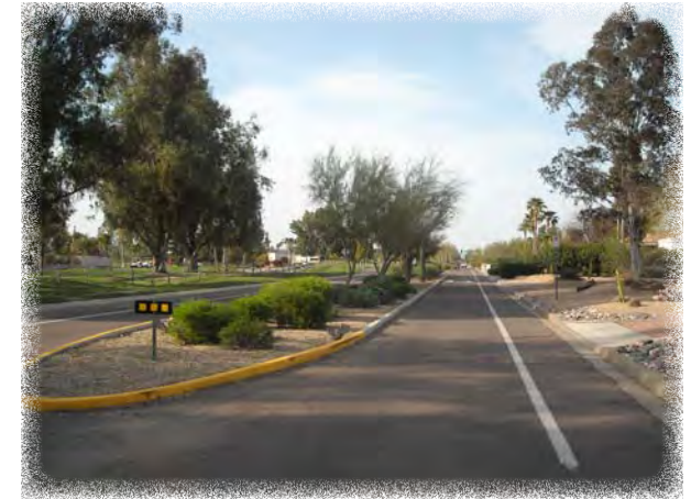
Bike lanes and a sidewalk on one side of the street help to keep this Scottsdale neighborhood's rural character while providing for multiple travel modes. Photo credit: Coffman Studio.
