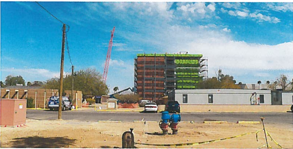
Context Photo 58 Looking East
