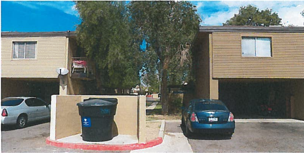
Context Photo 5 Looking North
