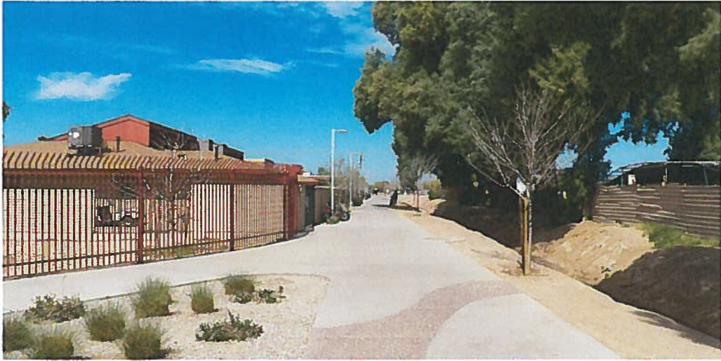
Context Photo 25 Looking North
