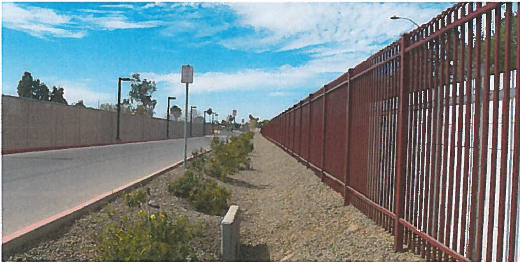
Context Photo 8 Looking West
