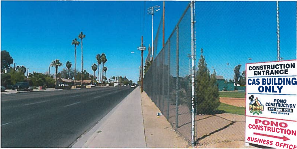
Context Photo 61 Looking North
