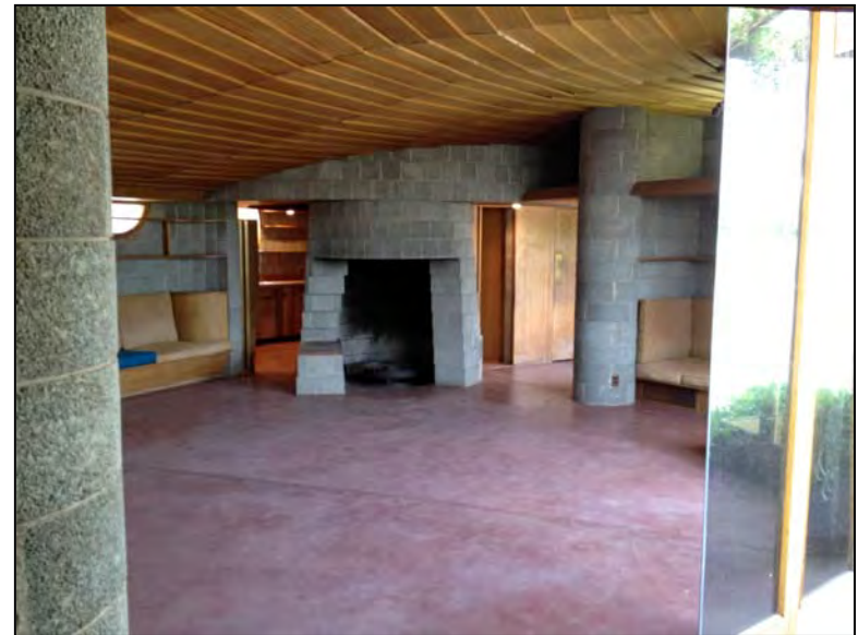
Photo 12. View of living room from bedroom wing
