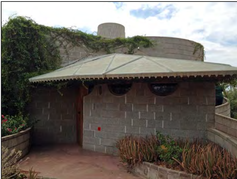
Photo 7. Main entrance to house at top of ramp
