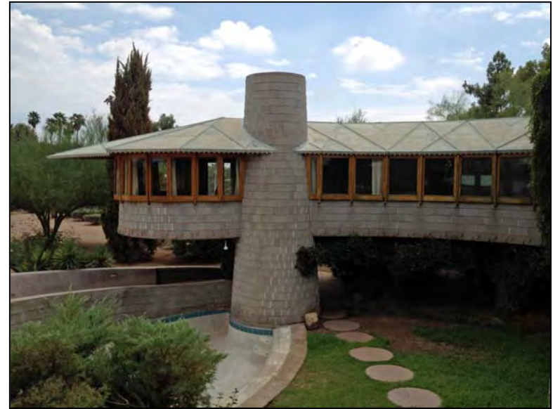
Photo 6. View of bedroom wing from ramp leading to second story
