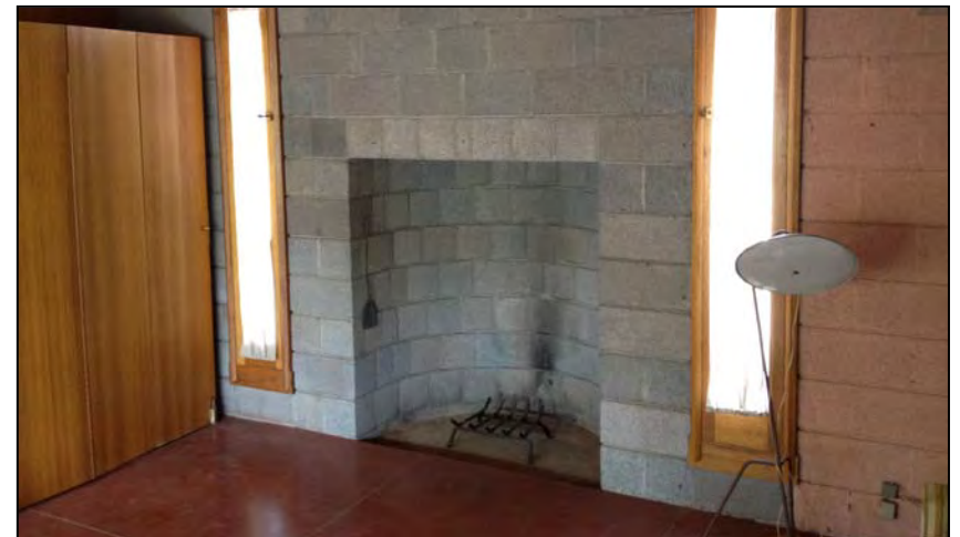
Photo 17. Guest house interior
