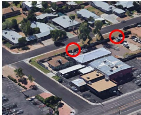
Openings in wall on Brill Street
