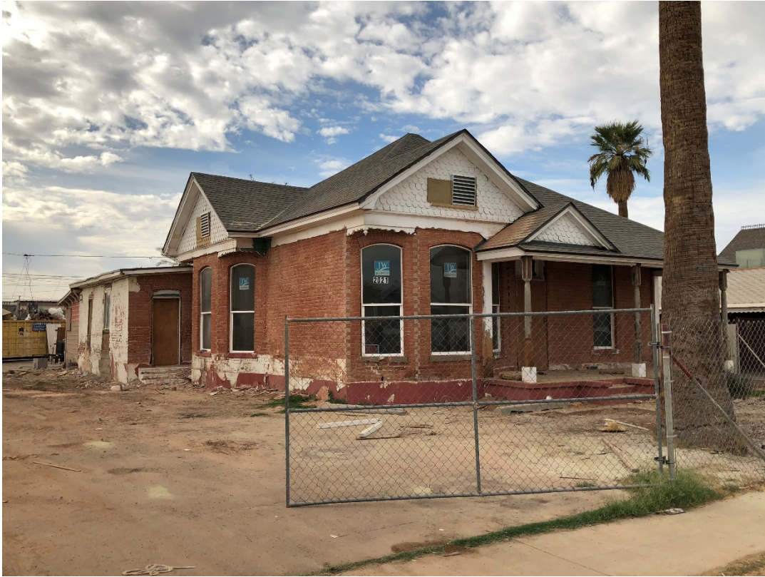
10/31/2017 – Front/side view, looking southwest from driveway
