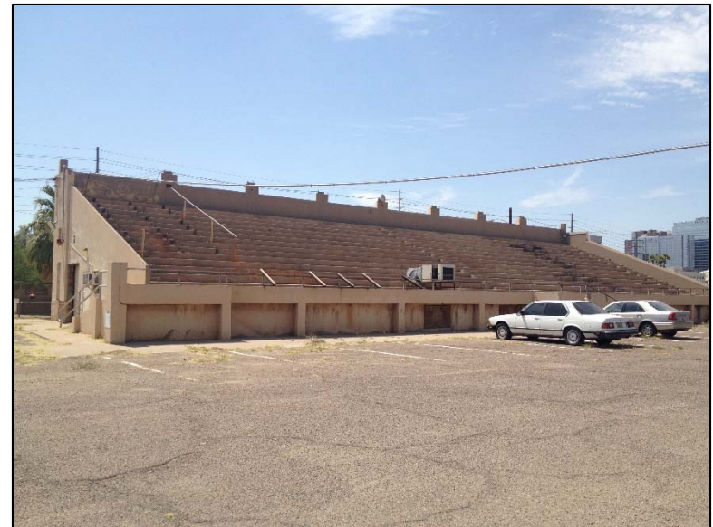
Photo 4. Concrete stadium at rear of property, looking northwest from rear property line.
