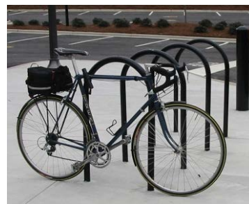
Inverted-U bicycle rack, where both ends of the "U" reach the ground.
