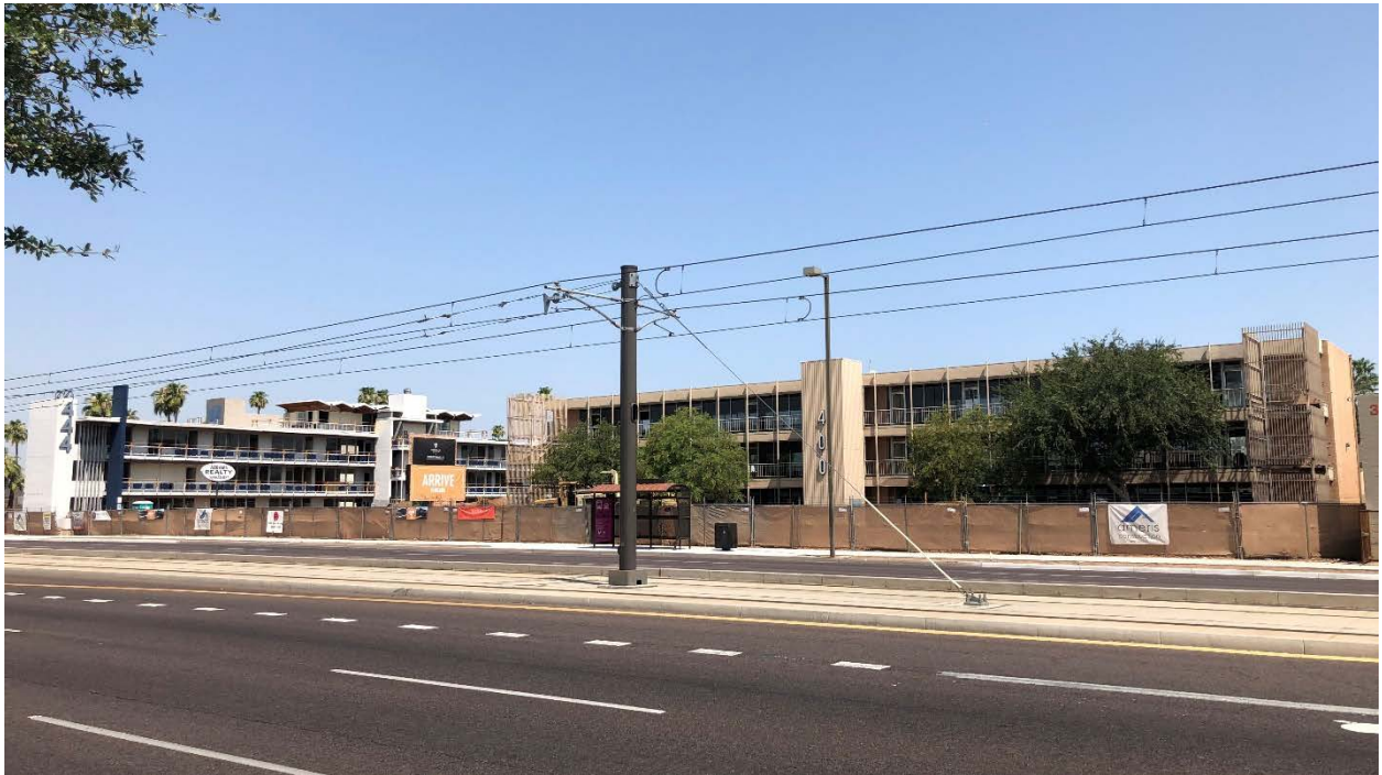
Photo 1. View of 400 & 444 West Camelback Road from opposite side of street, facing northwest. Rehabilitation is in progress (2018).
