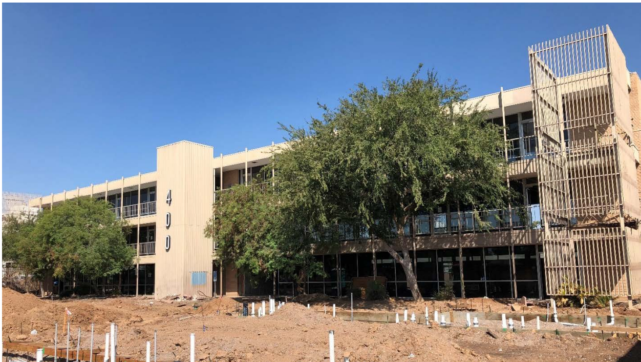
Photo 4. View of 400 West Camelback Road from inside construction fence, facing northwest (2018).
