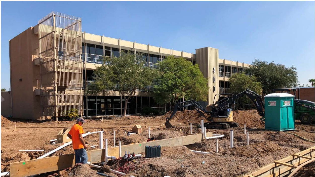
Photo 3. View of 400 West Camelback Road from inside construction fence, facing northeast (2018).
