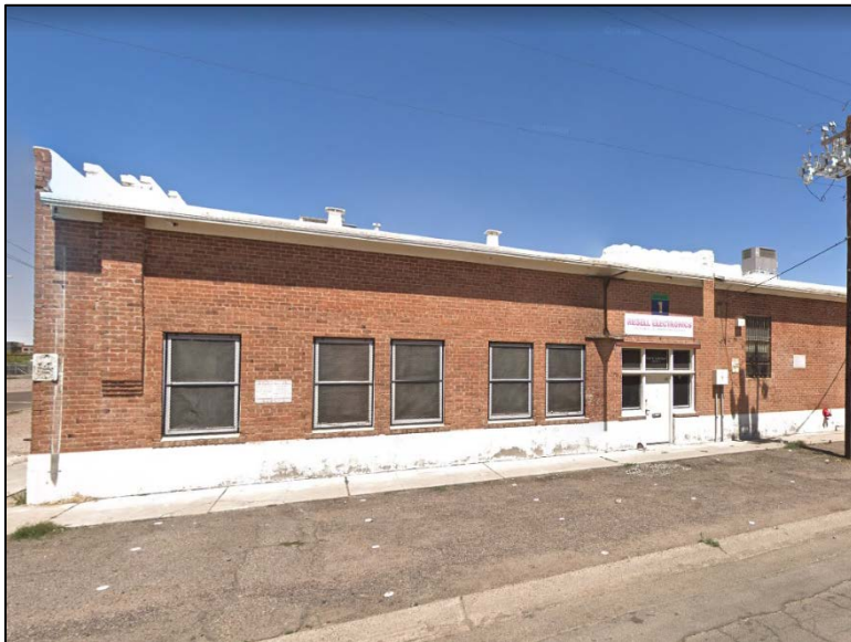
Photo 3. Exterior view of front office portion of 1927 building, looking north from Lincoln Street.
