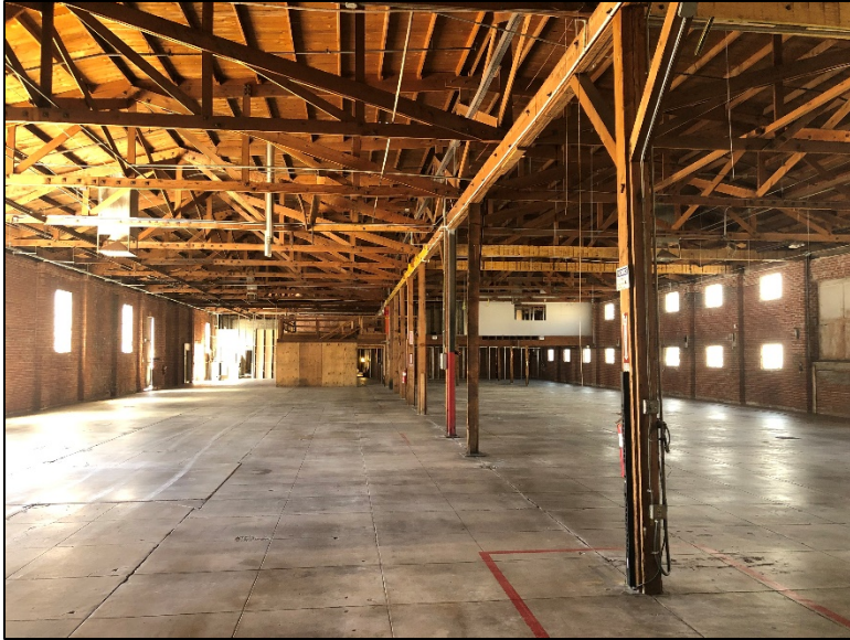
Photo 9. Interior view of warehouse portion of 1927 building, looking west.
