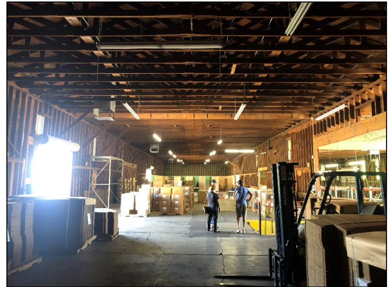
Photo 12. Interior view of encapsulated historic wood frame structure, looking east.
