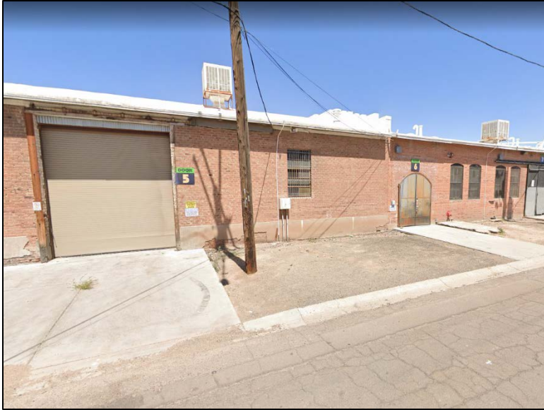
Photo 5. Exterior view of transition from 1927 building to 1943 addition, looking north from Lincoln Street.
