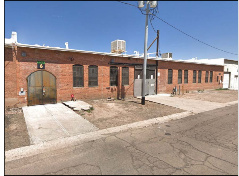
Photo 6. Exterior view of 1943 addition, looking northeast from Lincoln Street.
