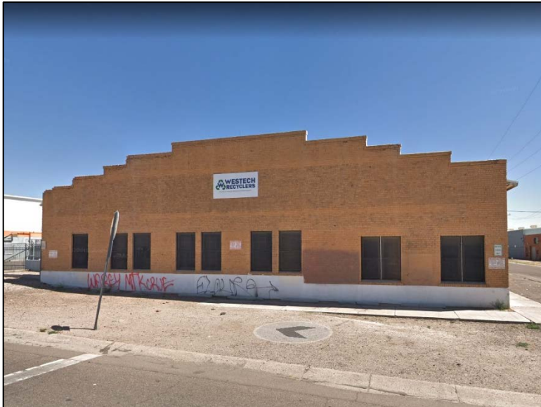
Photo 1. Exterior view of 1927 building, looking east from 9 th Avenue.
