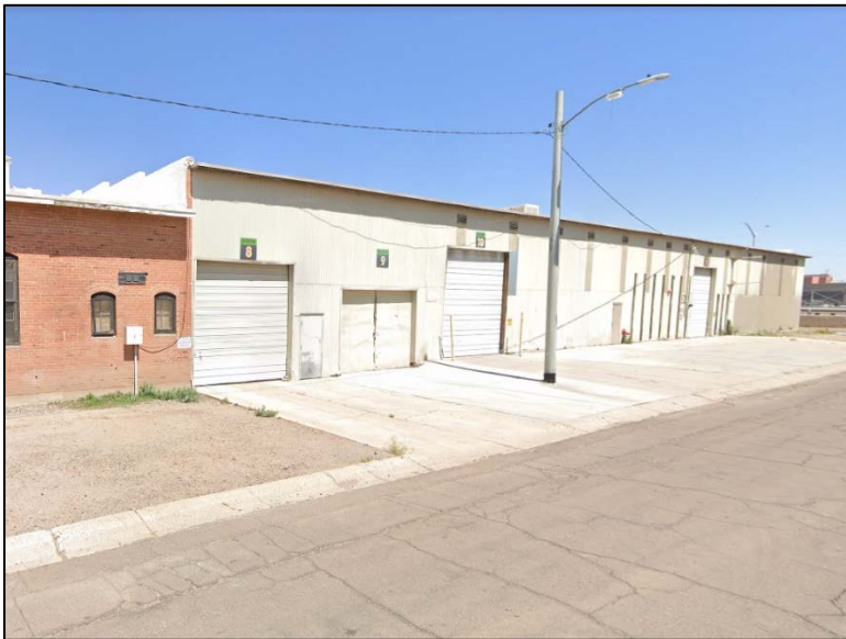
Photo 7. Exterior view of nonhistoric metal addition, looking northeast from Lincoln Street.
