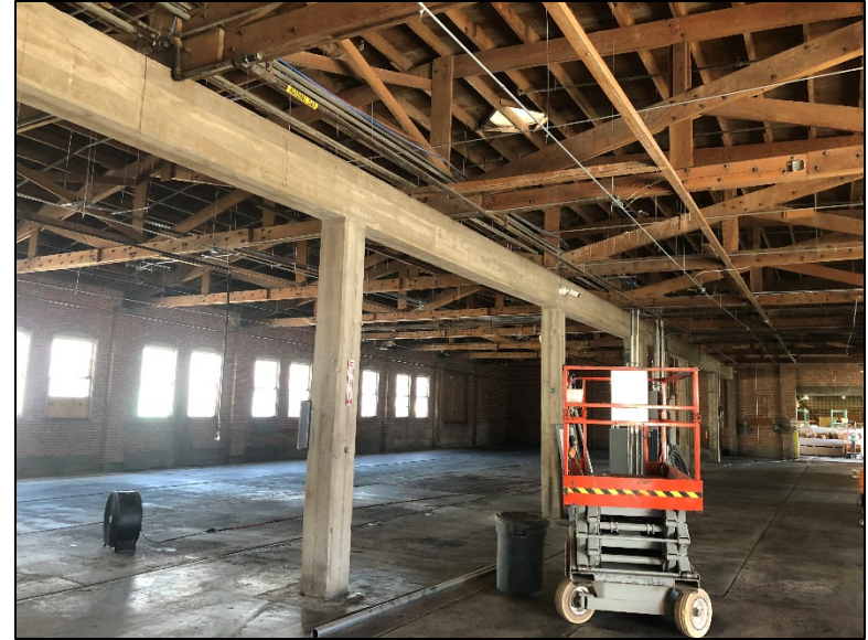
Photo 10. Interior view of 1943 addition, looking northeast.
