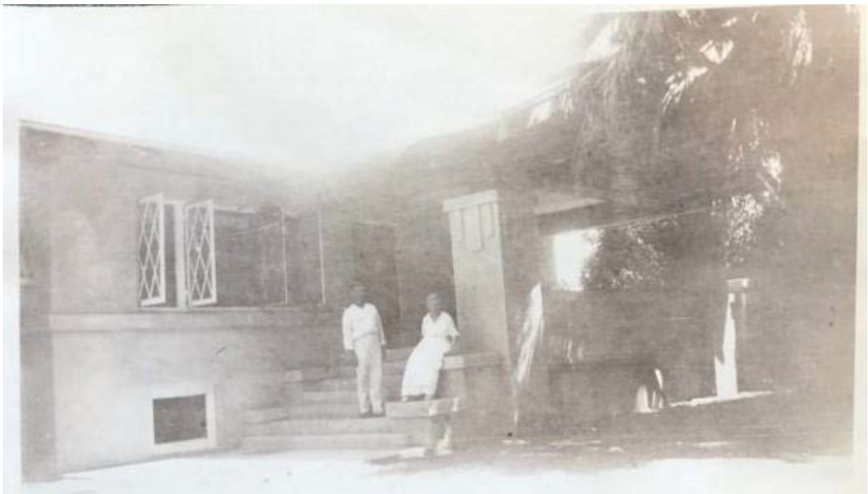
Frank & Emma Avery on the front porch of their house. Note the casement windows, stucco horizontal banding, stucco knee brace trim on the simple, square column.
