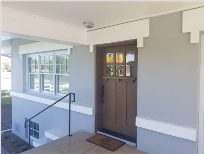
Photo 3. 4203 N 44th Street, front entrance.
