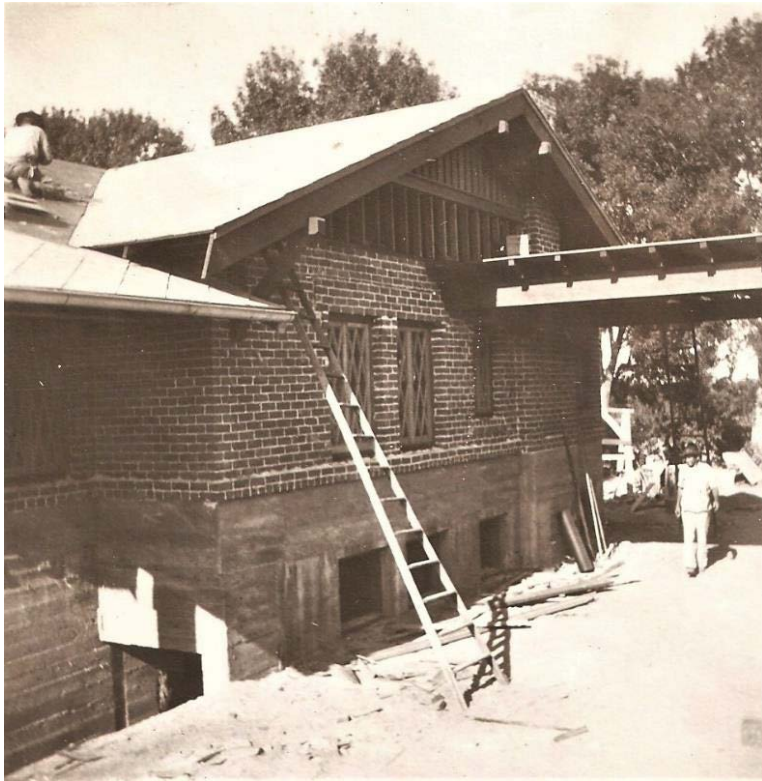
North side of house with the beginning of the porte-cochere.
