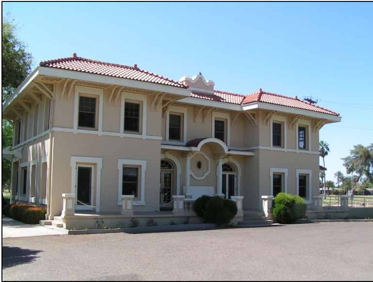
Photo 5. The Norton House, facing northwest.
