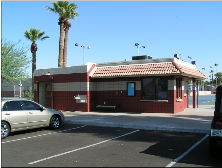
Photo 21. The equipment room of the sports complex in Side B, facing northwest..
