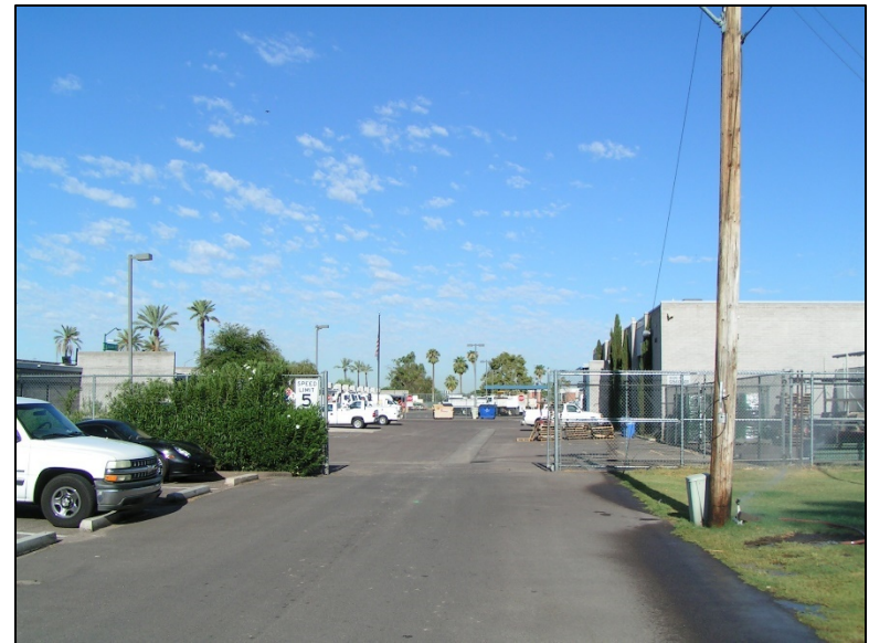
Photo 20. The east entrance of the maintenance yard, facing west.
