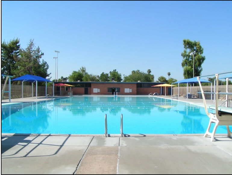
Photo 25. The swimming pools and bathhouse in Side B, facing south.
