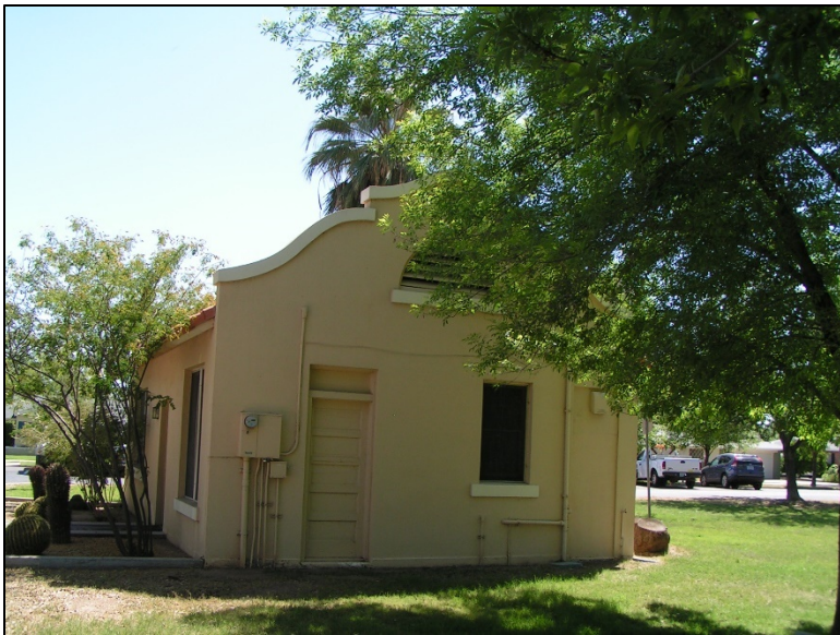
Photo 11. The Annex Building, facing southeast.
