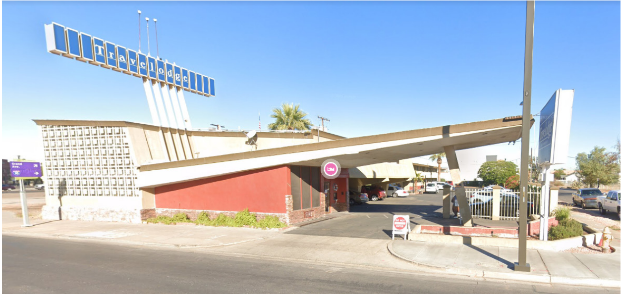
Main building, south view. Google image captured February 2020.
