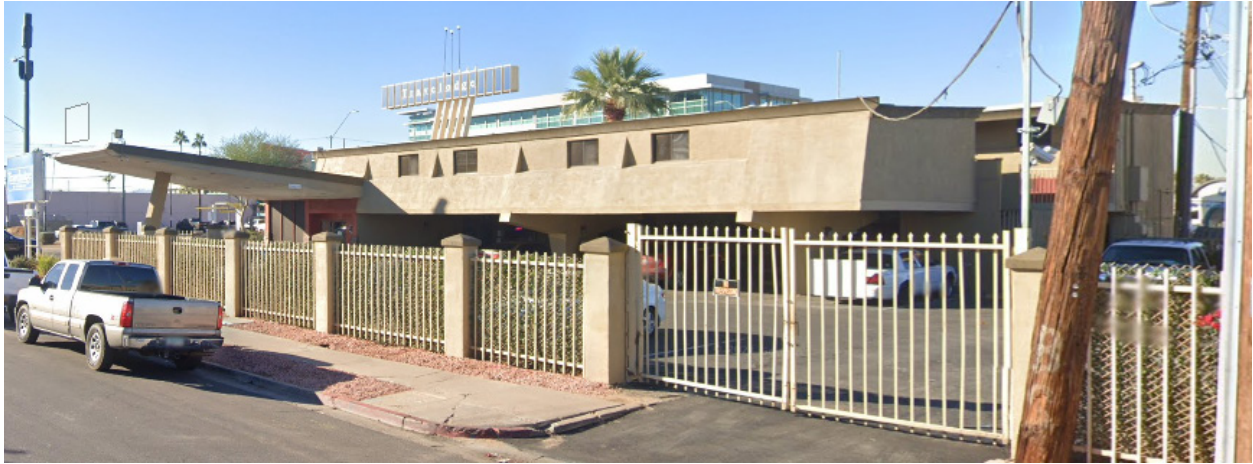
Main building, northeast view. Google image captured February 2020.
