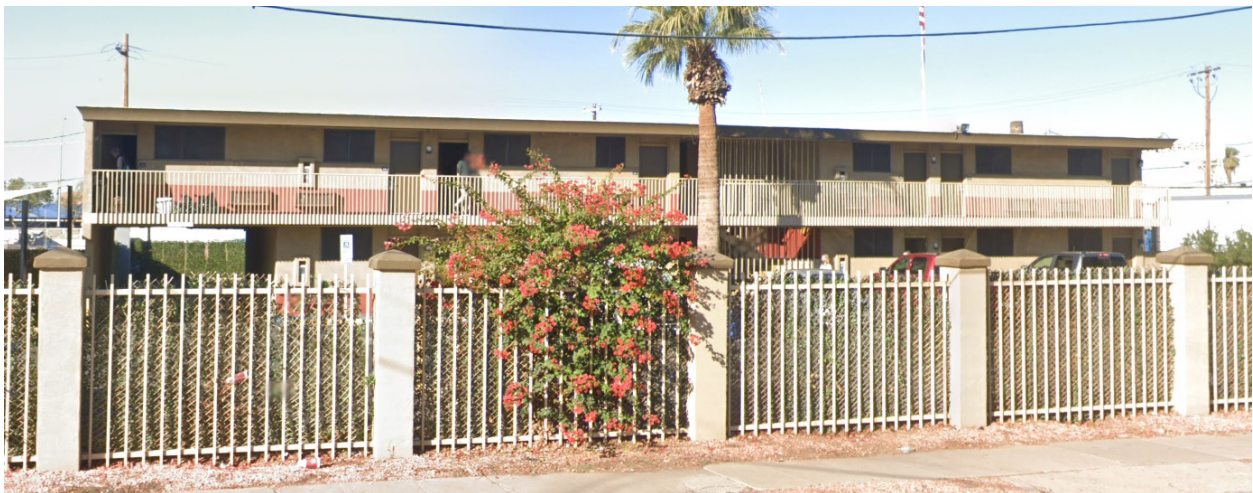
Annex building, east view. Google image captured December 2020.
