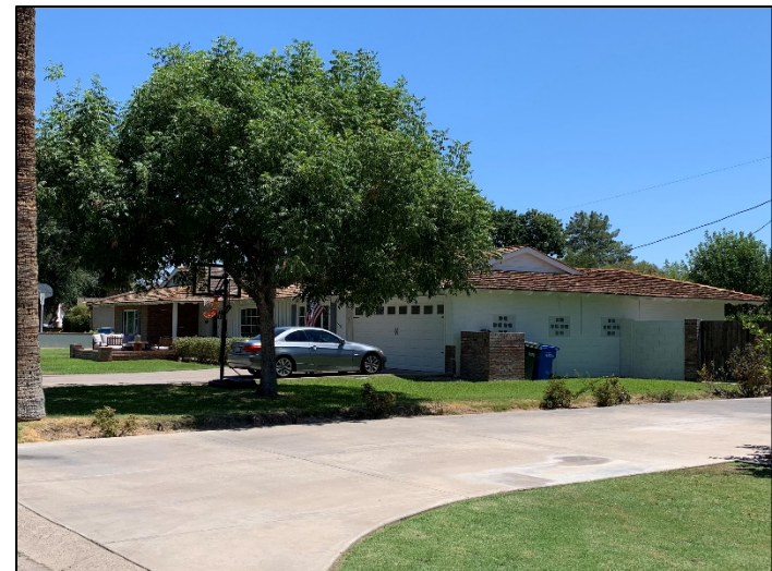
Photo 4. 333 W Gardenia Dr, looking southeast.
