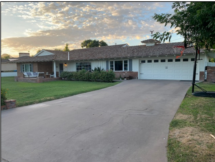
Photo 3. 333 W Gardenia Dr, looking southeast.
