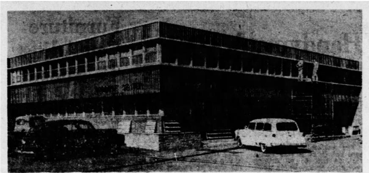
Building Completed The New Produce Center building, McDowell and 21st Ave., now is complete and practically filled with firms' associated in the vegetable growing and shipping business of Salt River Valley. It was erected by Ralph Eaton and features an interior landscaped patio, with balconies serving as halls to second-floor offices. Workmen on scaffold are installing aluminum sun louvers on upper windows. The overhang of the second floor shades the lower windows. Lester H. Laraway was architect.—(Republic Photo, Rod Moyer)
