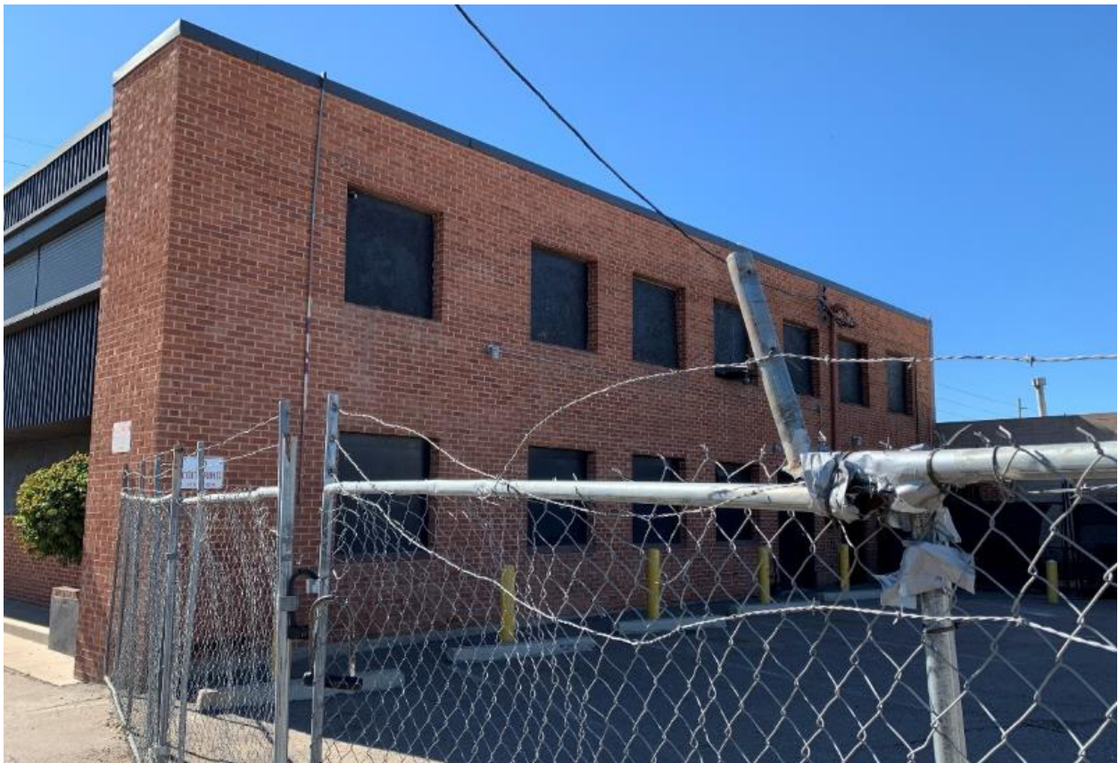
Northeast corner of building, looking southwest, January 2020
