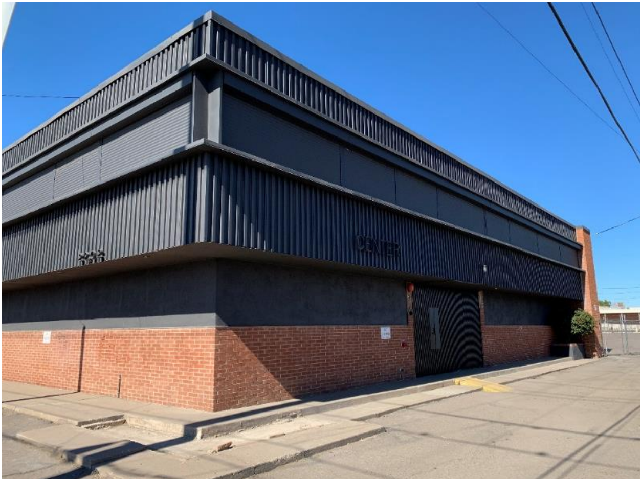
Southeast corner of building with gated entrance to interior courtyard located along eastern façade, looking northwest, January 2020
