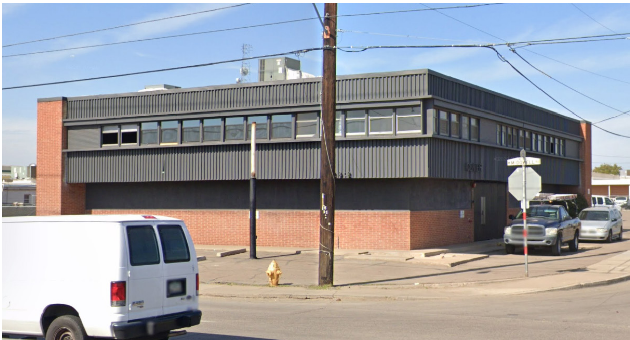
View of building with second story windows uncovered, looking northwest from intersection of 22 nd Avenue and McDowell Road, February 2020
