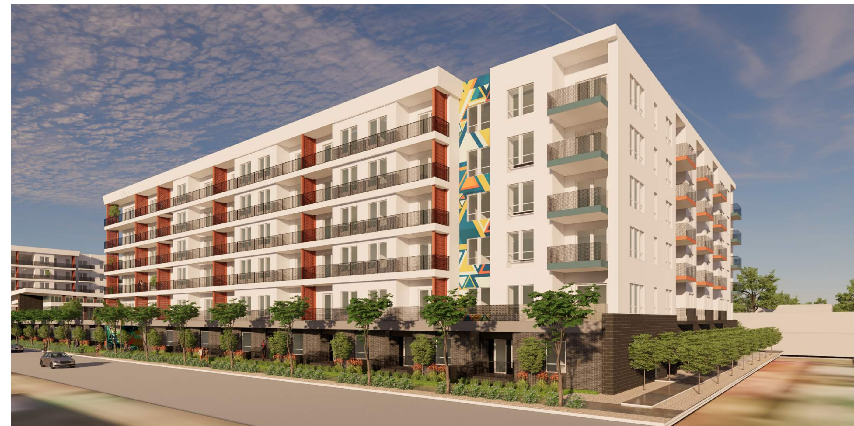
NE CORNER VIEW ALONG 4TH
