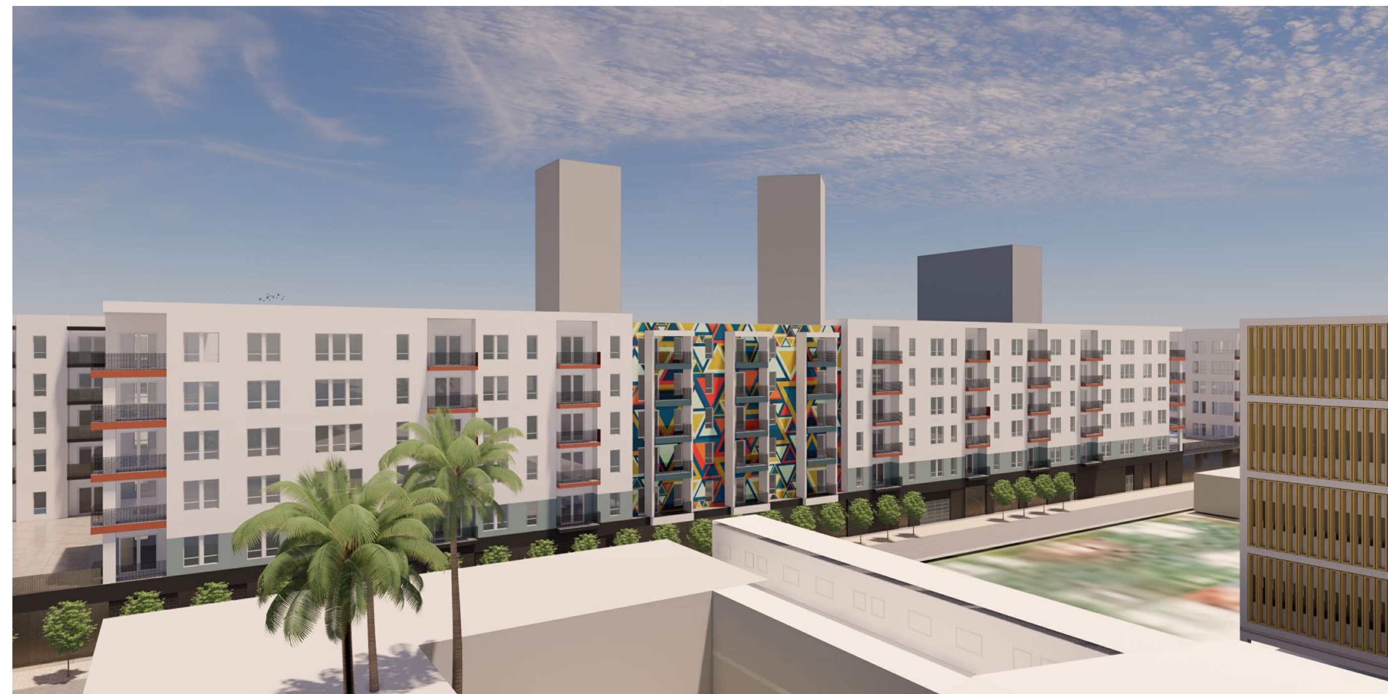
AERIAL VIEW ALONG ALLEY
