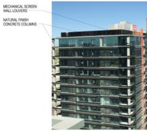
7 KIERLAND IMAGE, MECHANICAL LOUVERS 1/4" = 1'-0"
