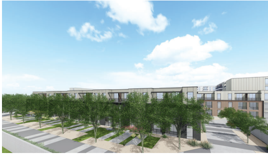
VIEW LOOKING NORTH
