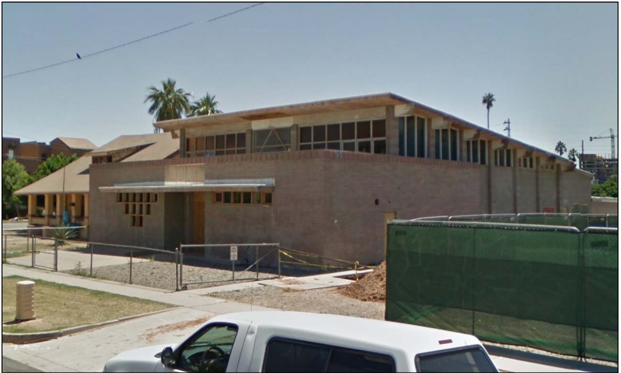
Photos of Beth Hebrew Synagogue in 2016 showing rehabilitation in progress
