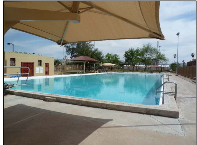
Photo 2. View of swimming pool, looking southeast from north end of pool.
