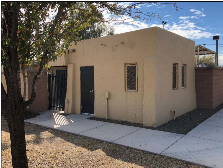
Photo 3. View of pump house, looking southeast from front lawn.
