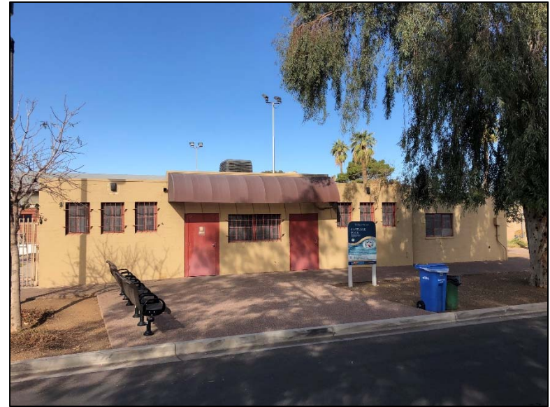
Photo 6. View of bath house, looking west from east parking lot.
