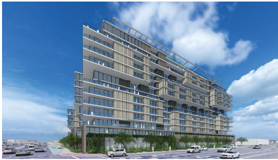
CORNER AT SCOTTSDALE ROAD + BELL ROAD LOOKING SOUTH
