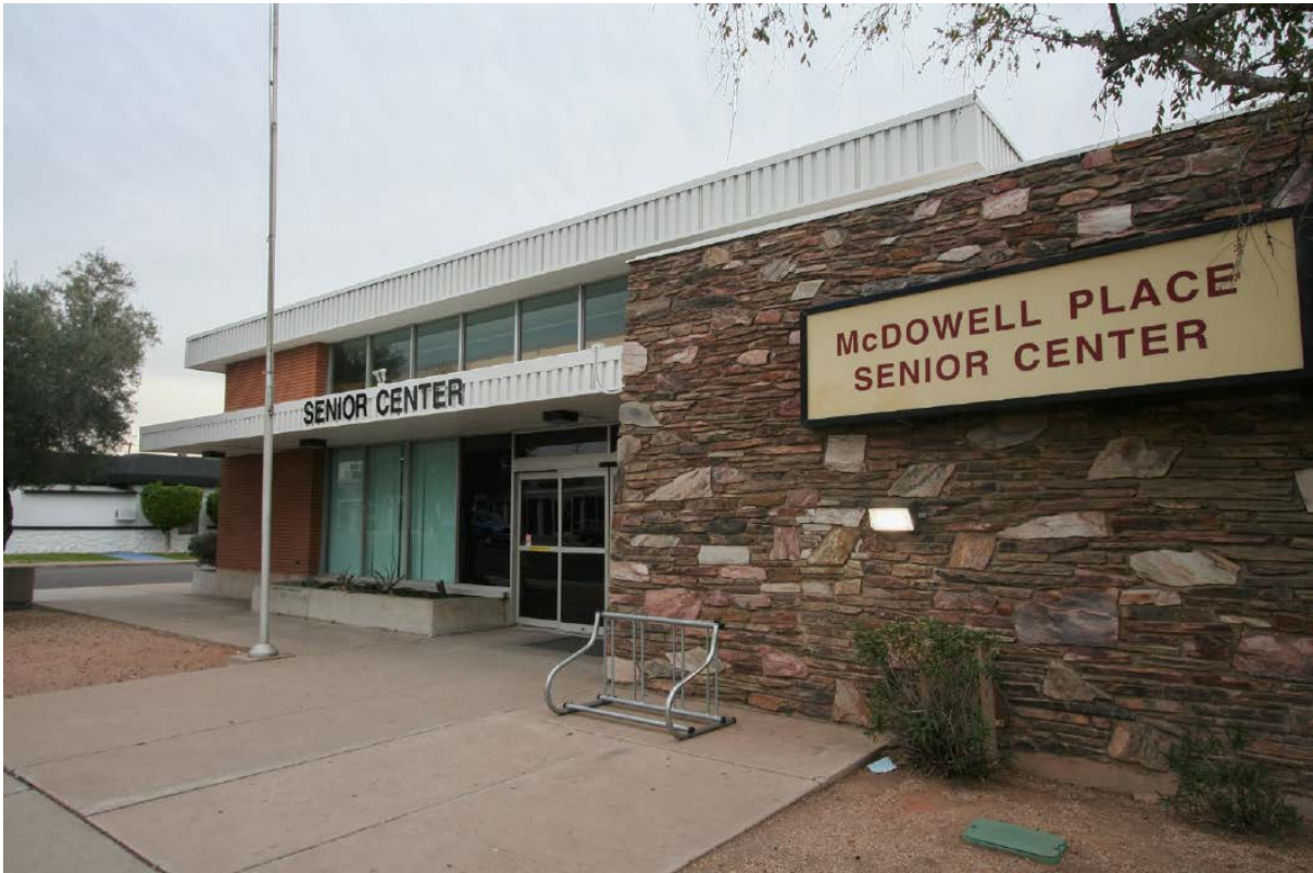
View looking southeast at north façade, December 2020
