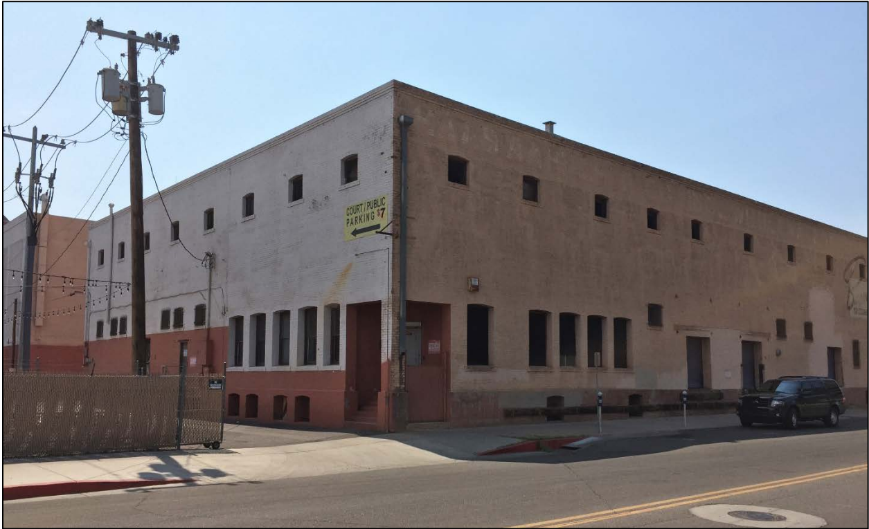
Photo 1. View of 1913 warehouse, looking southeast from 5 th Avenue, June 2017.
