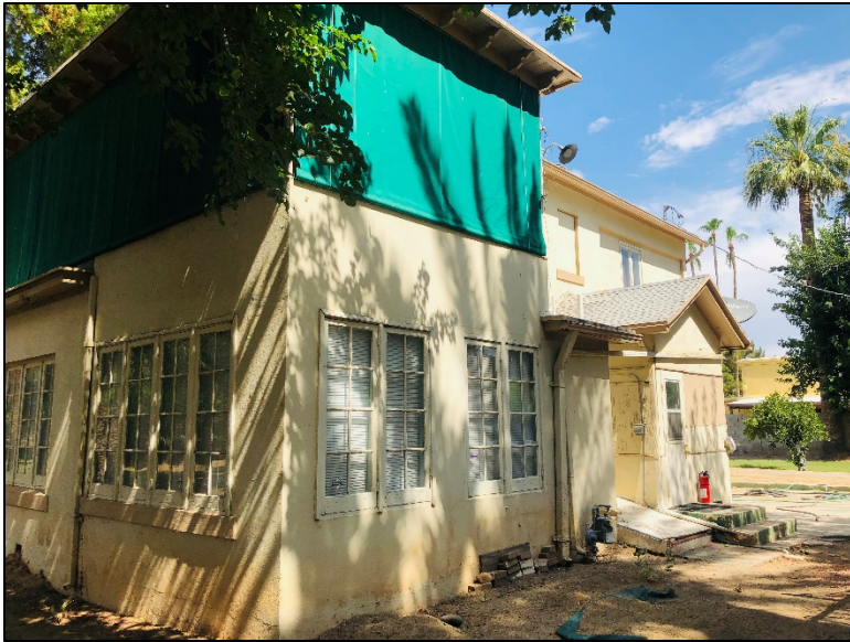
Photo 9. Close-up view of house, looking northwest from rear yard.
