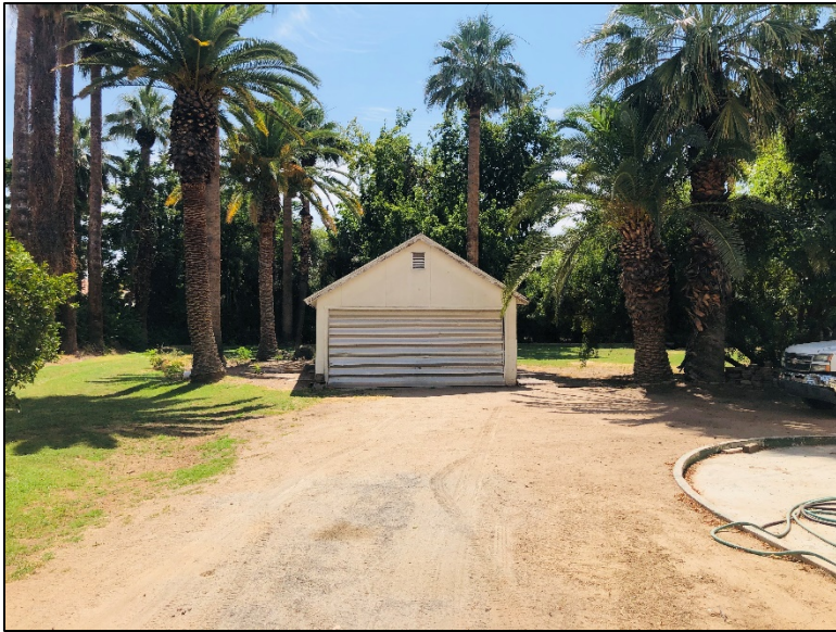
Photo 5. View of detached garage, looking east from circular driveway.
