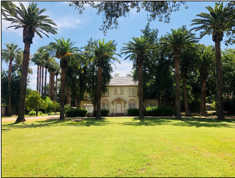
Photo 1. View of subject property, looking east from Murphy Bridle Path along Central Avenue.
