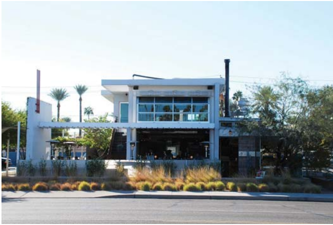
Adaptive Reuse - St. Francis Restaurant
