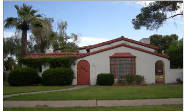
The front bay window of this historic house is a Tier 1 window and should be a high priority for preservation.
