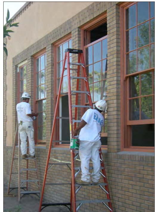
Historic wood windows at Steele Indian School Park are painted after being restored by a window repair specialist.
