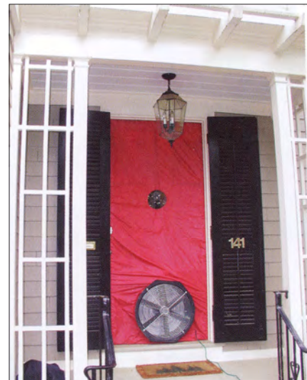
Energy auditors often use calibrated fans to measure the relative tightness of a building and to identify sources of air leaks.
