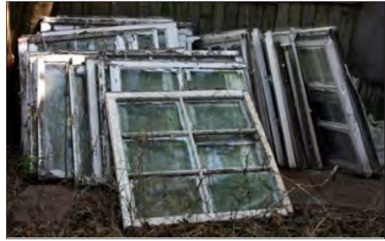
Removing repairable windows and dumping them in a landfill is contrary to “green” principles.
