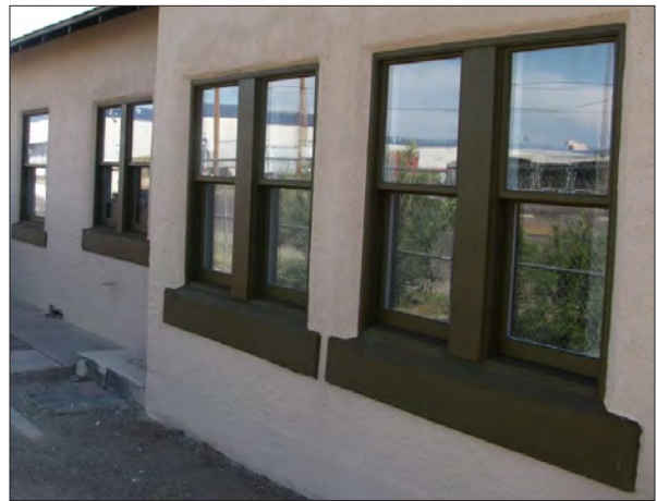
The replacement windows shown above illustrate the type of work that meets the "Recommended" requirements for both Tier 1 and Tier 2 windows.
