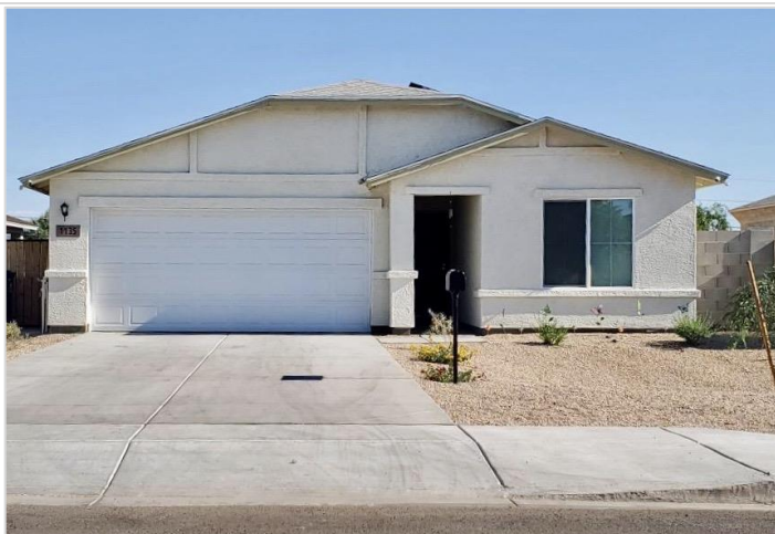
Habitat for Humanity, Matthew Henson Infill Project
